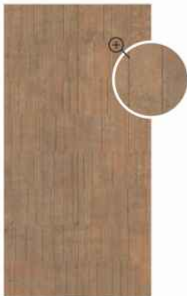
GROOVE IRON RUST
